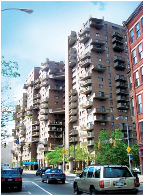
Andrews Terrace Apartments in Rochester, New York received repairs and improvements. (Photo courtesy of Rochester Downtown Development Corporation)
